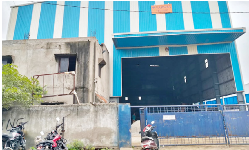
was granted, questions are being raised over how approval was issued if the construction dif-
