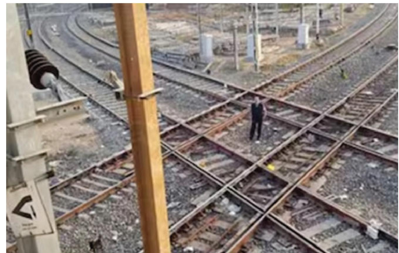
Nagpur Railway Station in Maharashtra is home to India's only Diamond Crossing, a rare railway junction where trains from four different directions intersect safely and seamlessly. This engineering marvel highlights the precision and efficiency of Indian Railways, ensuring smooth operations at one of the country's busiest rail hubs.
