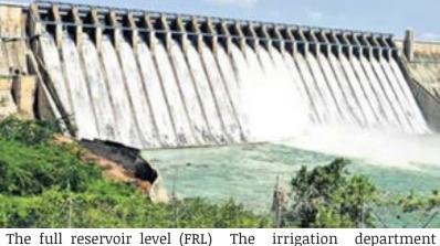
of Nagarjunasagar is 590 feet, while the current level stands at 586.5 feet, indicating a swift rise due to heavy upstream contributions. Out of the total storage capacity of 312.04 TMC, the reservoir currently holds 302.91 TMC, nearing its full potential.
